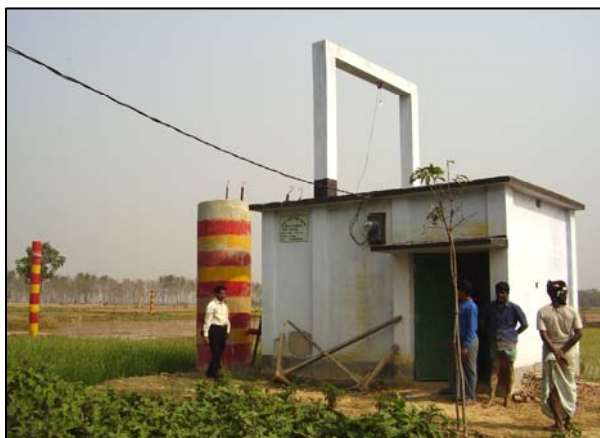
Installation of deep tube-well
